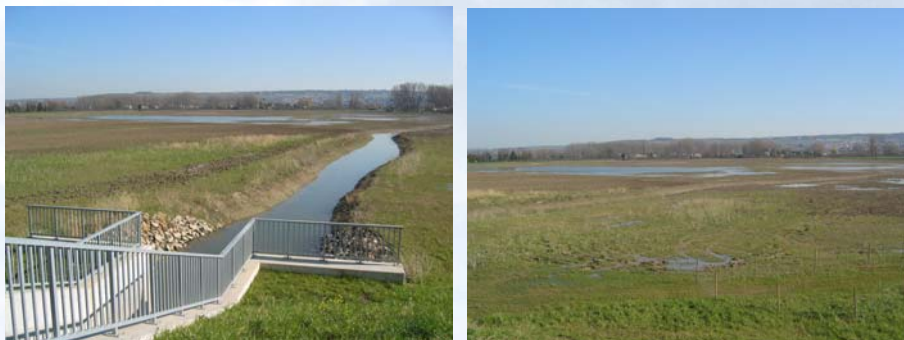
Inlet and area of ecological flooding
